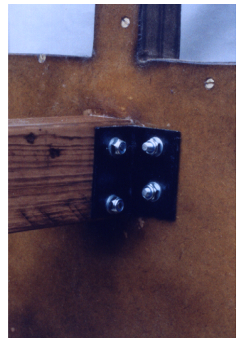
Angle bracket between stock and wheel
