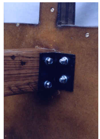
Angle bracket between stock and wheel
